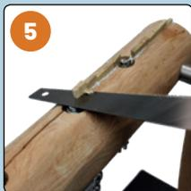
Saw off the protruding tops of the wooden wedges
