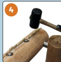
Hammer the wooden wedges into position
